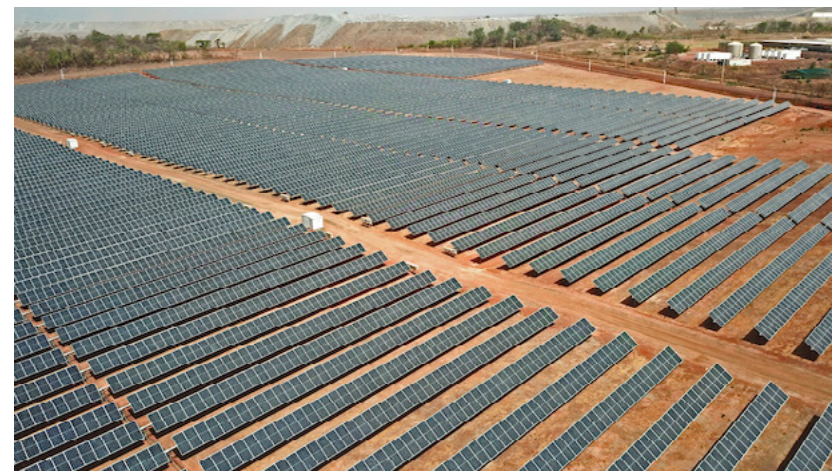
Onsite solar PV at Fekola gold mine in Mali, B2Gold Mining Company. Link to source
