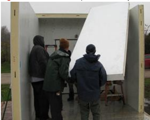
Figure 40. Insulated box panel assembly
