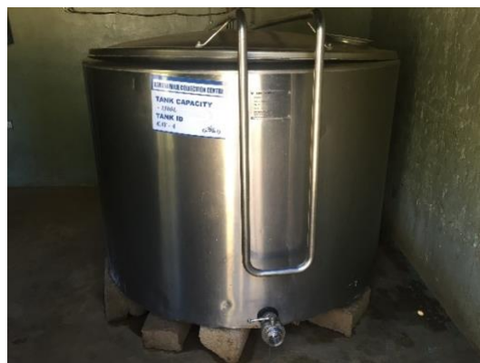
Figure 50. Example of a commercial collection point chiller
