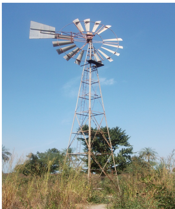
Figure 3.3: Typical Wind Pump System
