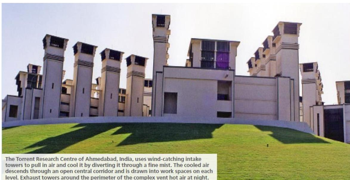
Figure 1 Example of an office building in Ahmedabad, India, using wind towers to naturally cool the building's interior<sup>ix</sup>
